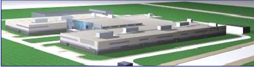
Three dimensional architectural rendering of the new manufacturing facility. The facility was designed in a “H-shape” with the two separate manufacturing wings and shared office, conference, laboratory and warehouse support space in the middle.
